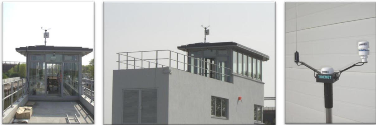
Figure 8 - TideMet Installation at Three Mills Lock
